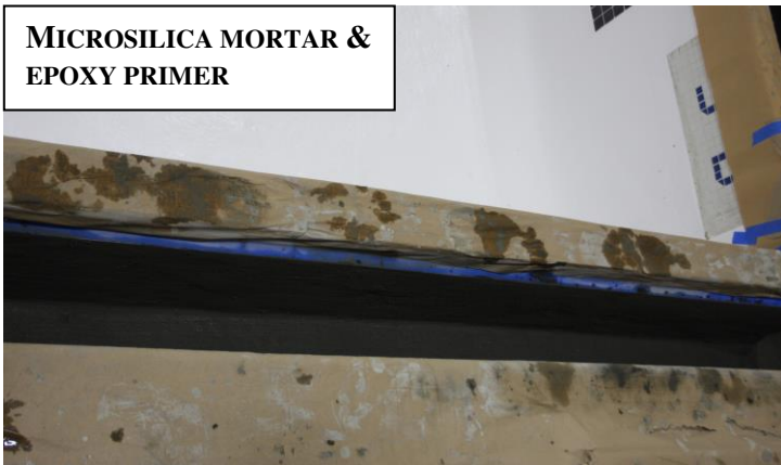
EPOXY AMINE SYSTEM COMPLETELY INSTALLED
