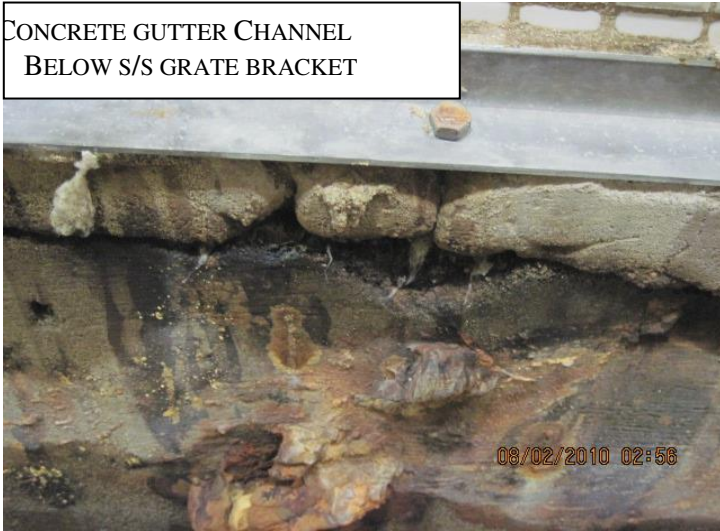
After High Pressure Water Jetting
