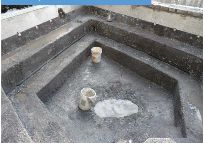
Gutted Spa to Sound Concrete Base
