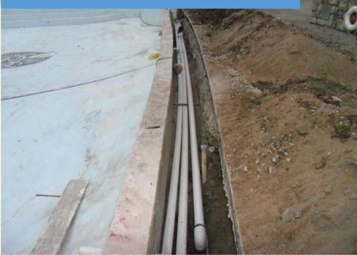
New Recirculation Lines in the Trenches
